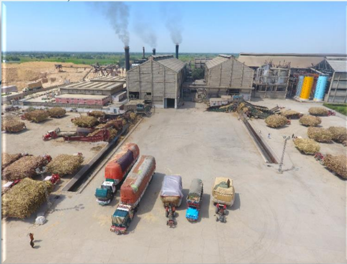
Chashma Unit – 1 Crushing Capacity: 12,000 MT/day
