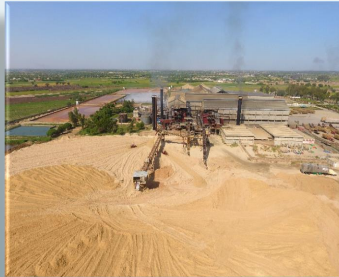
Chashma Unit – 2 Crushing Capacity: 6,000 MT/day
